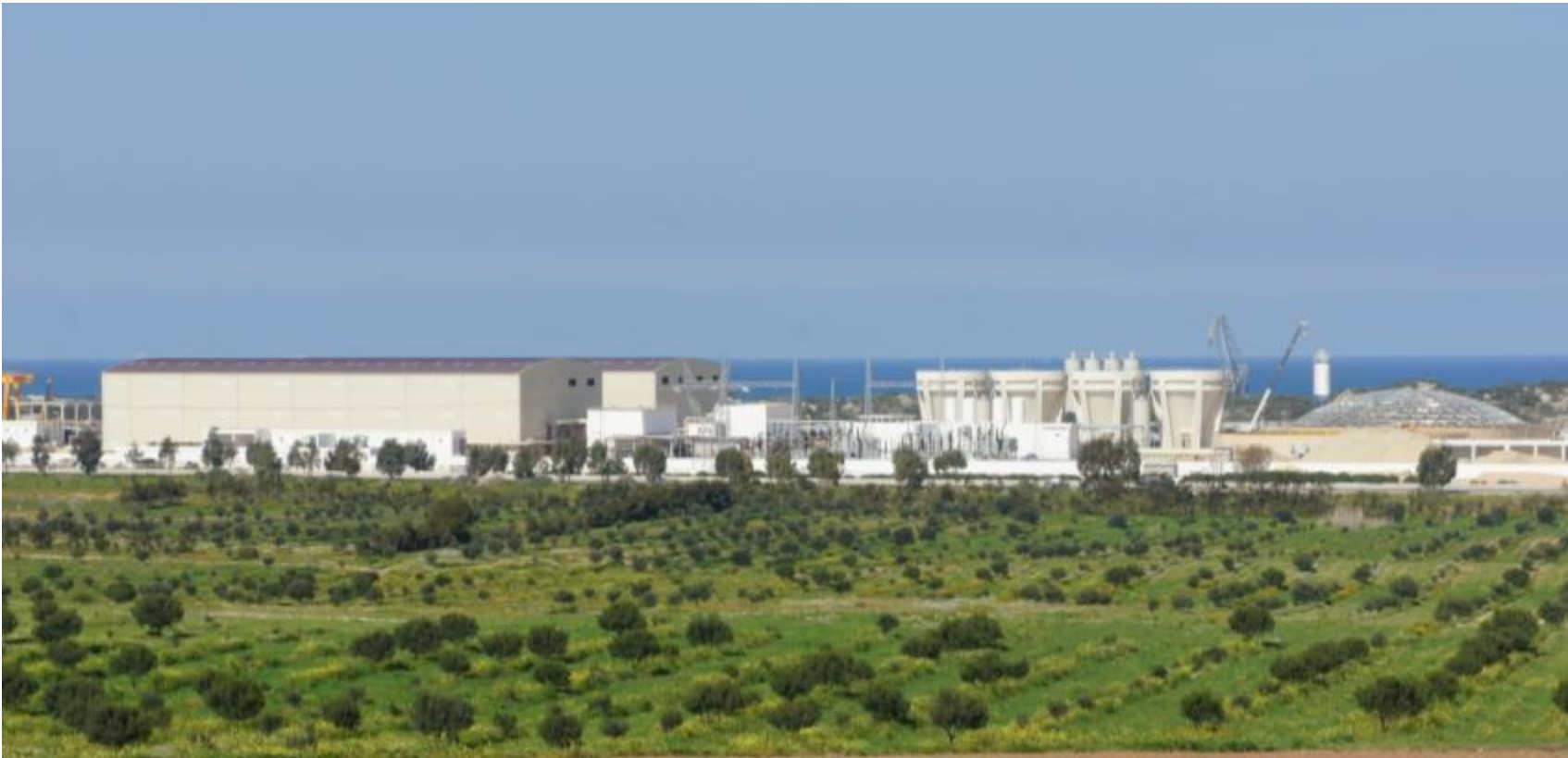
Overview of Magtaa Desalination Plant, Algeria
